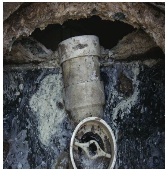
Left-Concrete Riser with MIC. The attack causes concrete to change to soft white Gypsum, which looks and feels like mashed potatoes.
