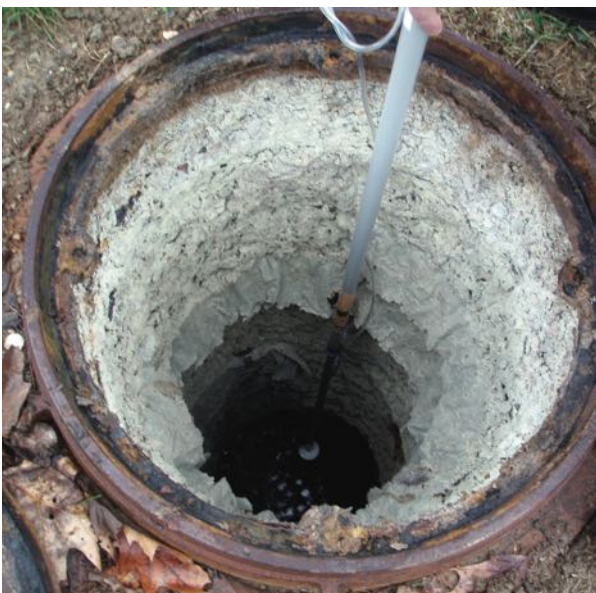
Left-Concrete Riser with MIC. The attack causes concrete to change to soft white Gypsum, which looks and feels like mashed potatoes.
