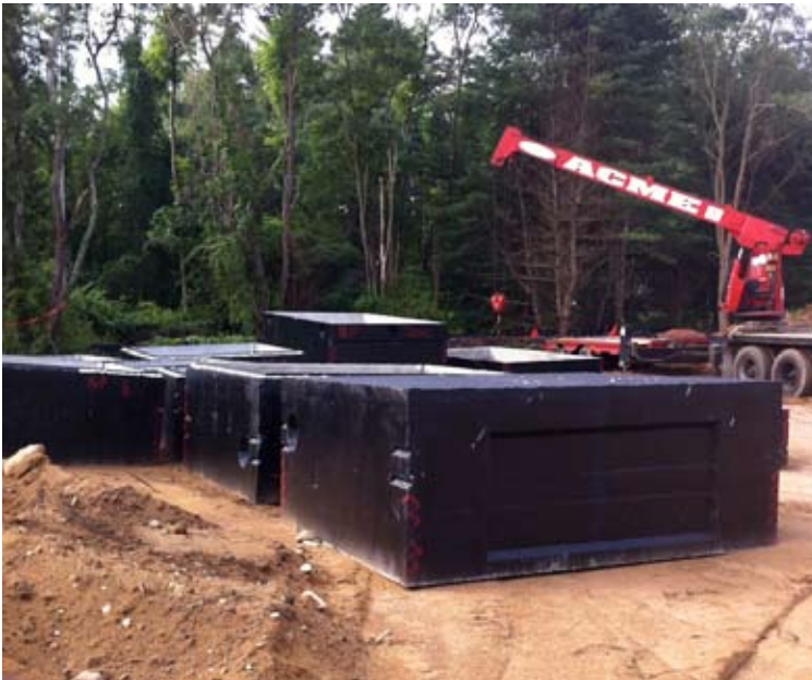
Acme's truck carries sections from the staging area to the crane.
