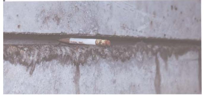
Dry fit your structures and visually inspect the joints on a regular basis. This septic tank joint was cast in a brand new form! The other end of the tank was so tight you couldn't slide a piece of paper in!
