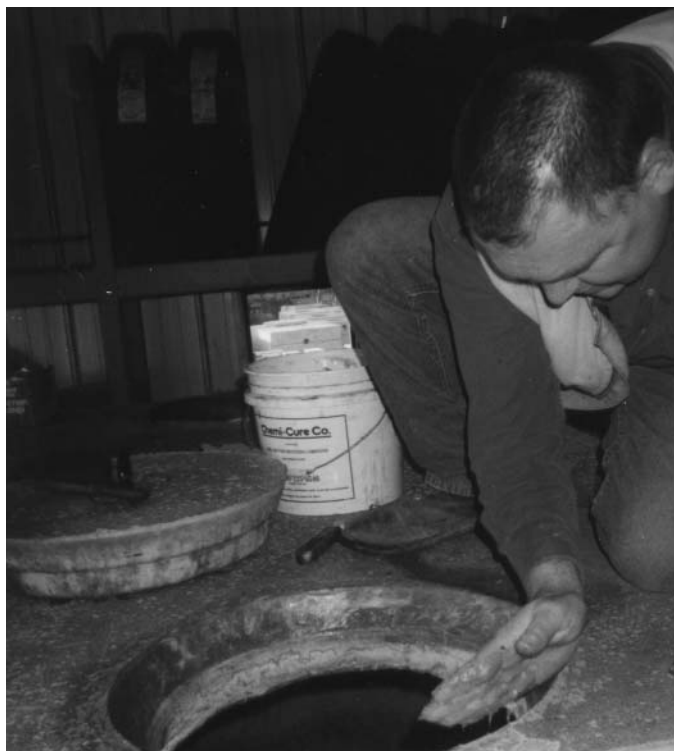
Dennis Jolley routinely vacuum tests his septic tanks. He smears tire lube on manhole cover.
