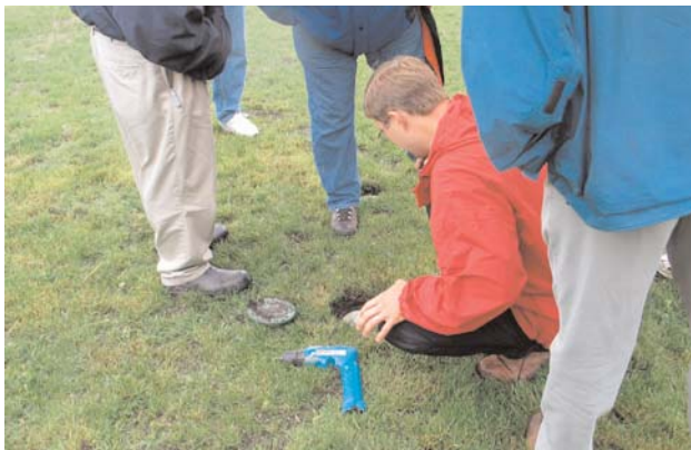
Accessible inspection ports allow monitoring of the shallow drainfield's performance in the lakeside onsite system.
